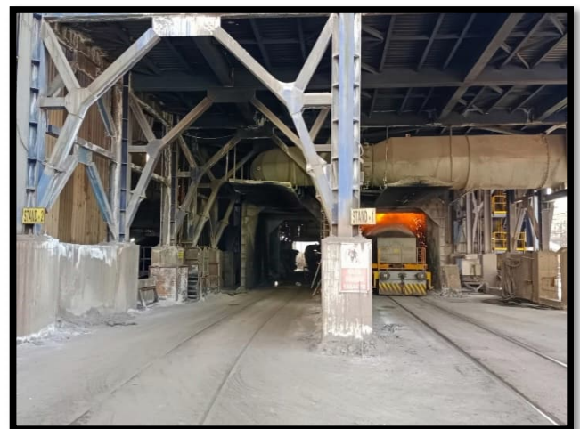
Figure 3. Blowing process being performed on liquid pig iron in a torpedo at desulfurization facility where studies were conducted.
